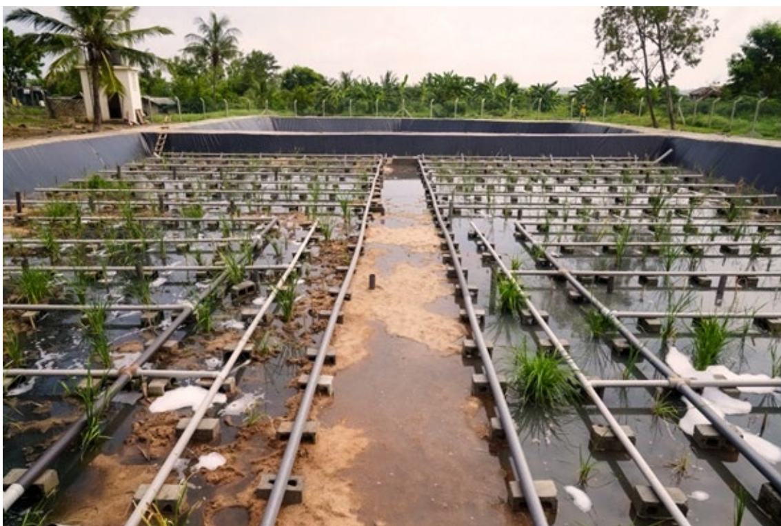
Figure 8: Constructed Wetlands Mimicking natural purification processes, these systems require minimal energy input whilst remaining highly adaptable to the unique conditions of informal settlements. Plants and microorganisms work together to break down contaminants.
