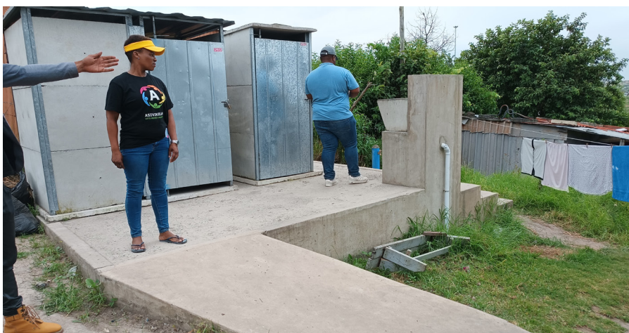
A Communal waterborne flush toilet in the Hani Park informal settlement in Buffalo City in 2024. The toilet has a wheelchair ramp and one of the toilets is suitable for use by persons with disabilities. The toilets can lock from the inside and is well-maintained. There is a basin with a tap, and an additional communal standpipe which is installed with the toilets.
