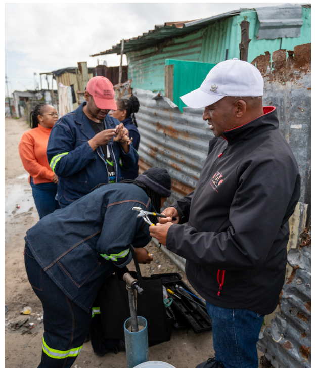
An Asivikelane community plumber in Cape Town replaces a missing tap on a standpipe in their settlement during a site visit.
