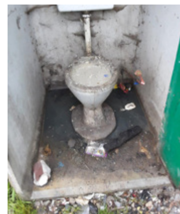
Block 6, Browns Farm (City of Tshwane)
