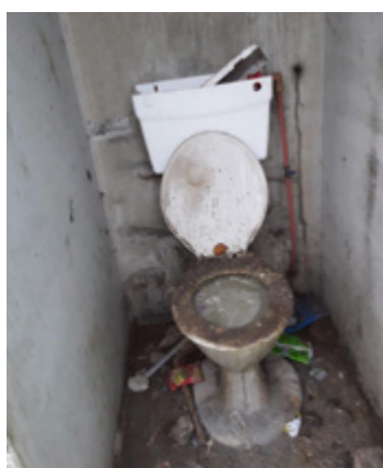
Block 6, Browns Farm (City of Tshwane)
