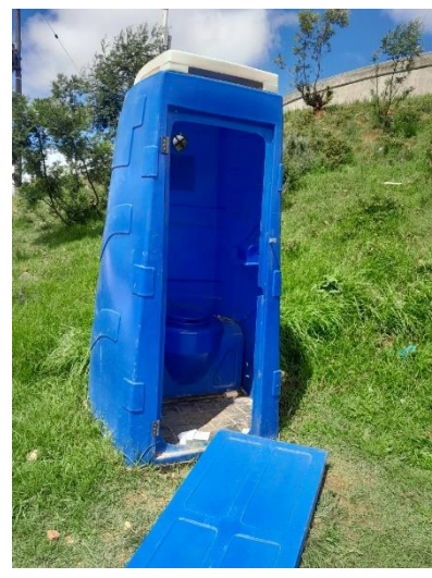
Figure 2 Toilet in Victor Molosi, broken door
