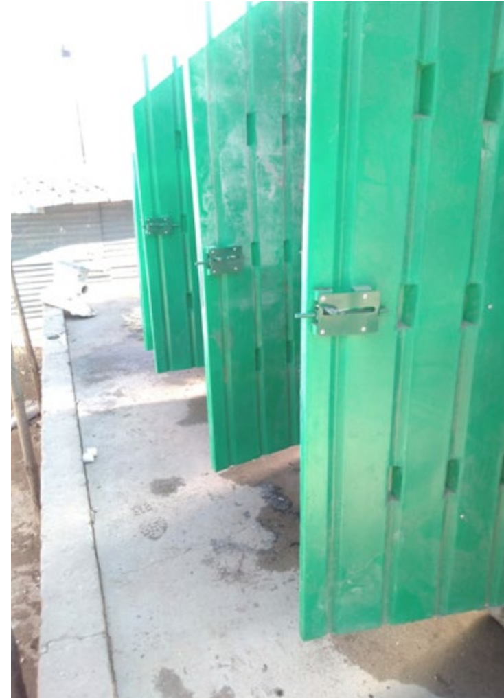
More than 50 toilets have been repaired in Langrug
