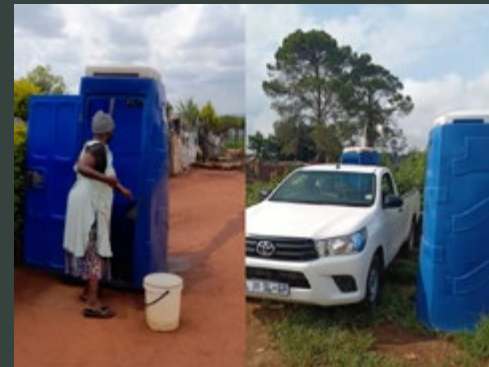
GOOD NEWS City of Tshwane Toilets were cleaned, drained and fixed
