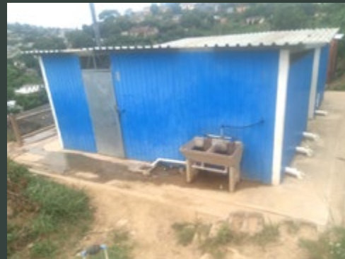
GOOD NEWS City of eThekweni Drains cleaned and unblocked and taps fixed
