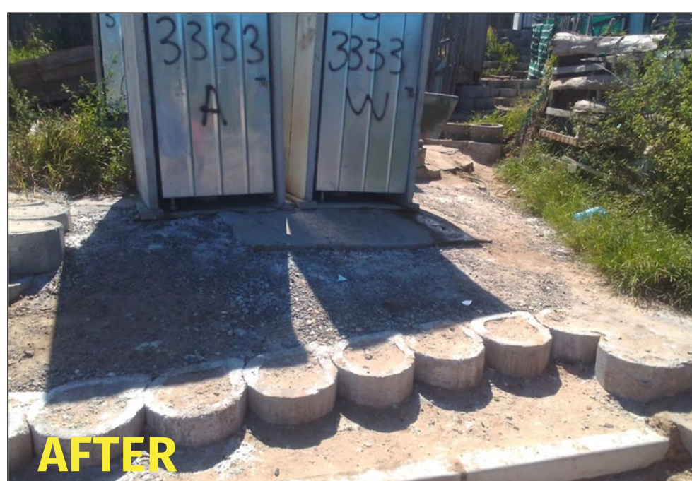
Toilet foundations paid for and fixed by the municipality in Smutsville.
